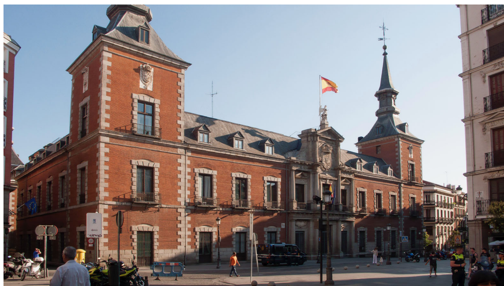
Figure 5. Cristóbal de Aguilera, Palacio de Santa Cruz, formerly Cárcel de Corte, 1629–40, view of the main façade with eighteenth-century reforms. Photo: Pablo Linés.
